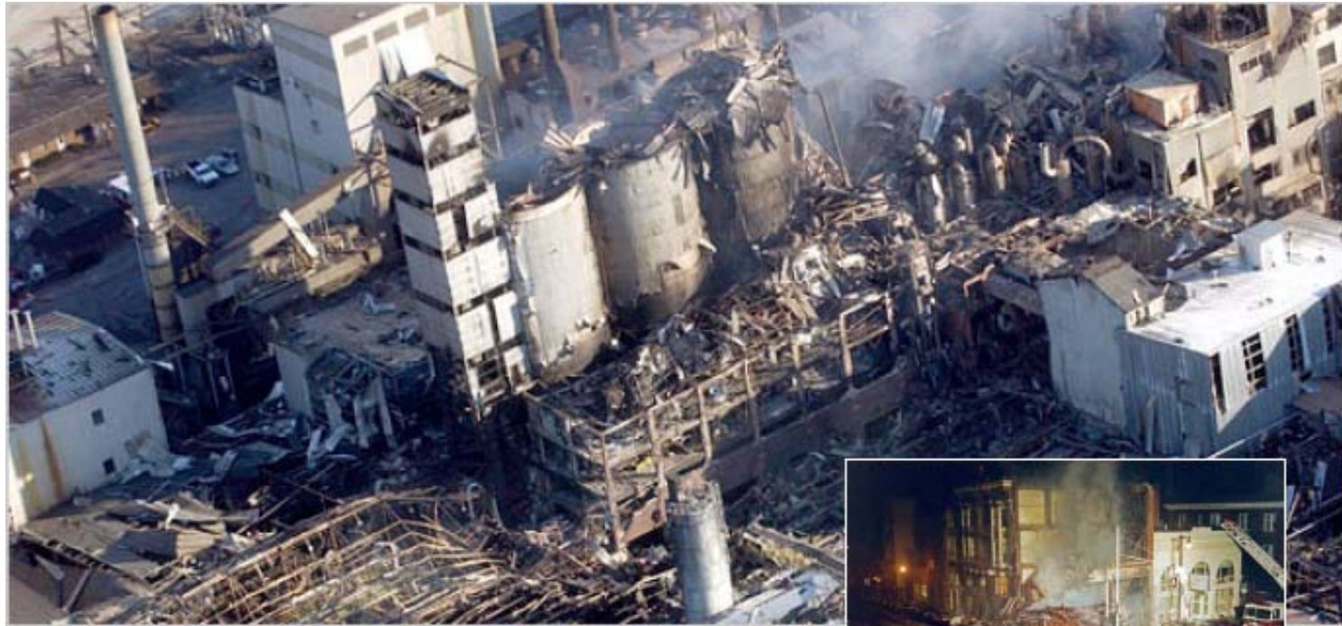
Devastating effects of a combustible dust explosion.
